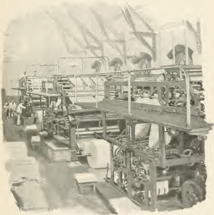
Three American-built Quadruple Presses Used by a Manchester Daily Newspaper
